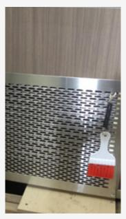
to regularly wipe away dust. Too much dust will not allow the refrigeration to work properly and could result in damage.
