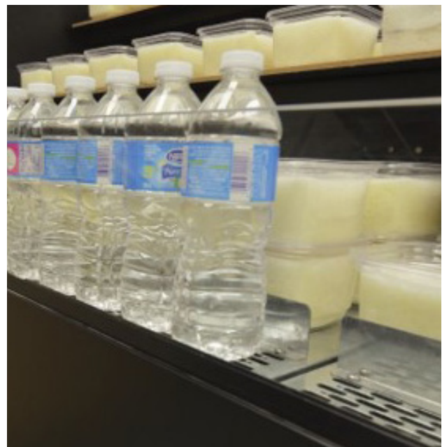
Blocked Air Vent
